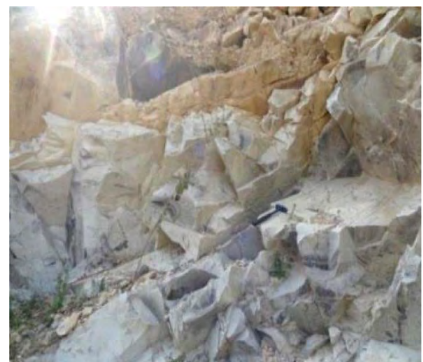
Figure 2: Joints Trending in E-w Direction in Felsite In Mogarahalli
